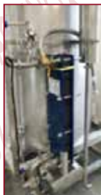
PLATE HEAT EXCHANGER
